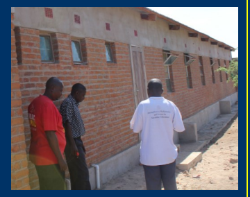
CHW Project Committee members inspecting completed hostel.
