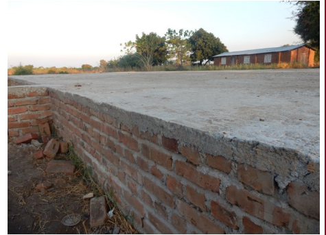
Brickwork is laid, cement was purchased and used to build foundation for a hostel for girls in Thunduti
